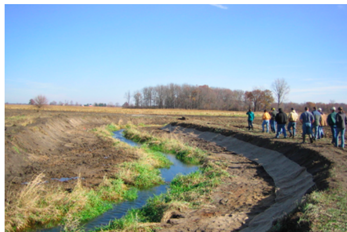
TWO-STAGE DITCHES CAN REDUCE FLOODING UPSTREAM
